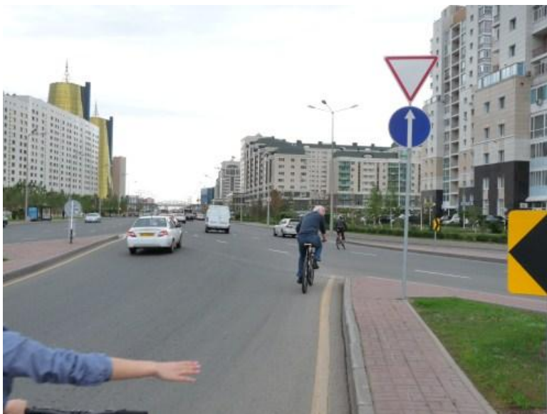
Fig. 7 Weaving is one of the most dangerous maneuvers. Traffic systems that are designed for high speeds and an undisturbed flow of motorized traffic, such as here at this merging of roads in Astana, lead to very dangerous situations for cyclists (and also for other motorized traffic).
